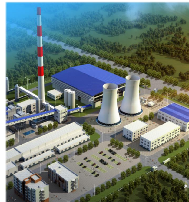
潍坊滨恒热电联产项目供热工程 3×240t/h CFB Boiler+2×B30MW
