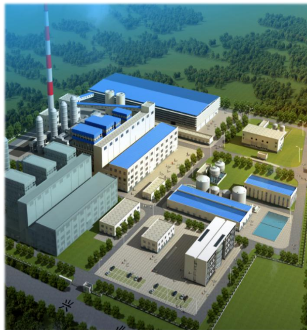
威海市经区桥头热电工程 2×35t/h CFB Boiler+2×B3MW
